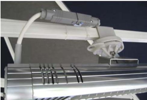
Secure cable by means of cable ties in the area of the heat transmission unit and make sure that it does not interfere with a possible pivoting movement.
